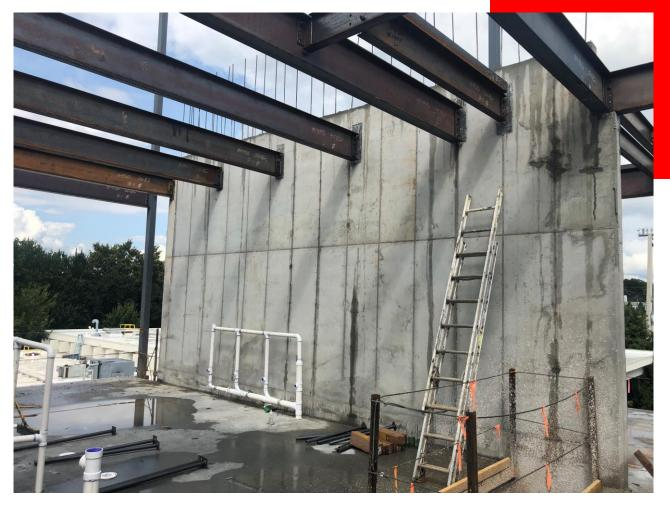
4<sup>th</sup> Floor Steel Tied Into New Shear Wall
